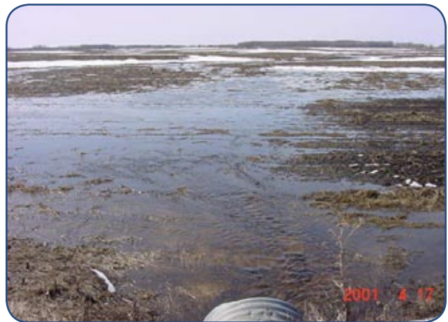
Typical runoff sampling site at discharge end of culvert.
