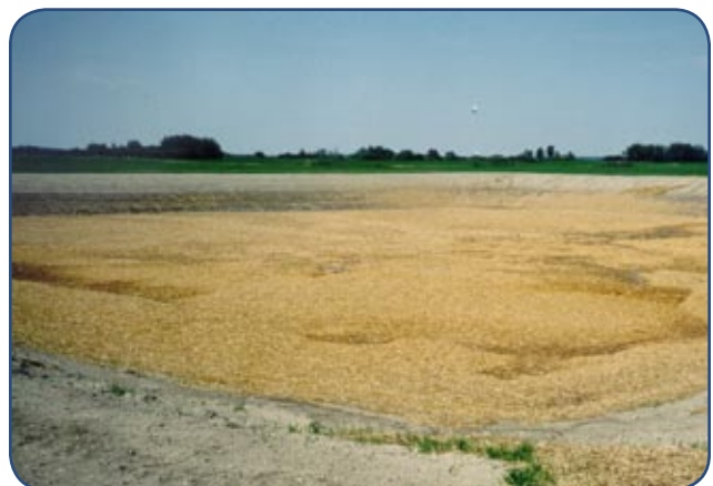
Straw covered earthen manure storage.
