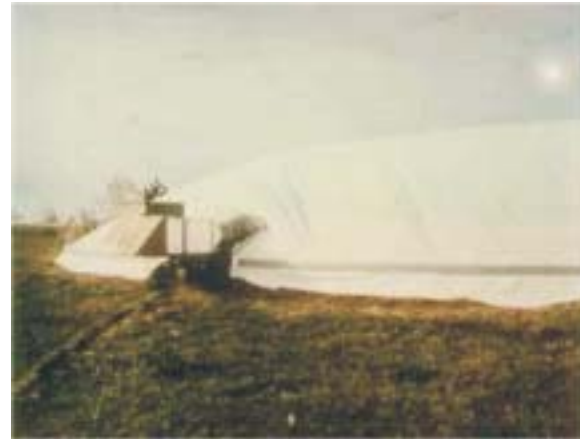
Synthetic manure storage covers shed rainwater and reduce nutrient losses.
