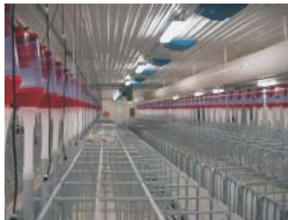
Vapour proof 4 ft fluorescent fixture. Photo Courtesy: Agviro Inc.
