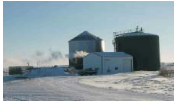
A biodigester in operation. Photo Courtesy: Clear-Green Environmental Inc.
