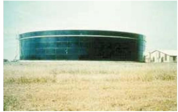
Steel storage structures for some locations where the subsoil is very coarse.
