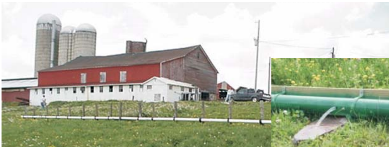
Vegetative filter strips (VFSs) treat runoff through infiltration, settling, absorption, and aeration. Photo Courtesy: Canadian Pork Council
